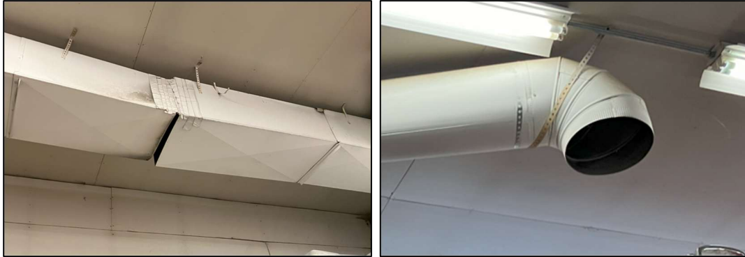
Area where ductwork improvements should be made (left), ductwork without terminal diffuser (right)
